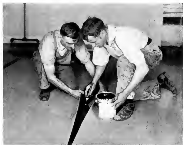
APPLYING CEMENT TO THE FELT
